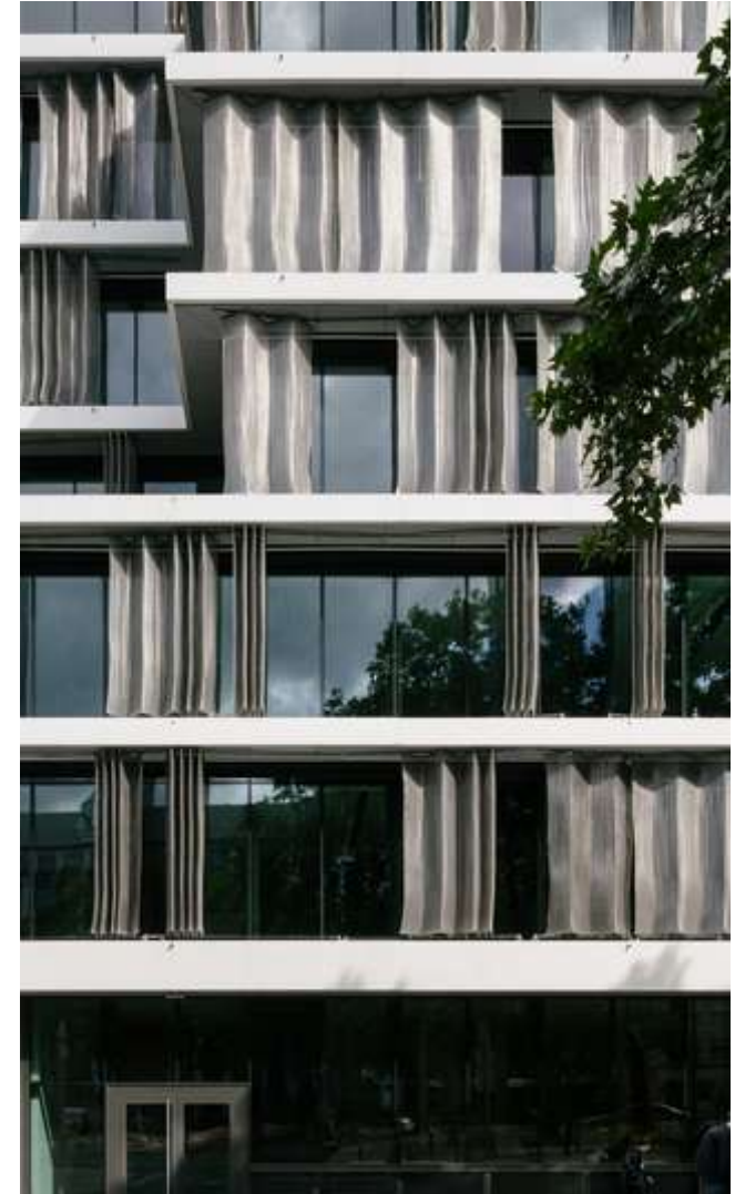
► Office building Quartz - Brussels' CBD (BE)
