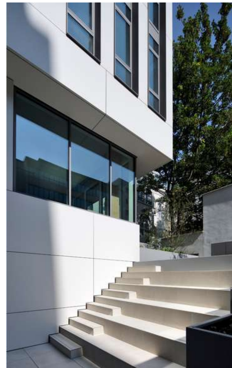
► Office building Montoyer 10 (M10) - Brussels' CBD (BE)
